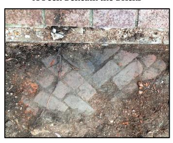
Recently the town conducted some major repairs on a section of sidewalk in front of 304 Mill Street. Tree roots had buckled the sidewalk to a point where it was no longer safe for pedestrians.
